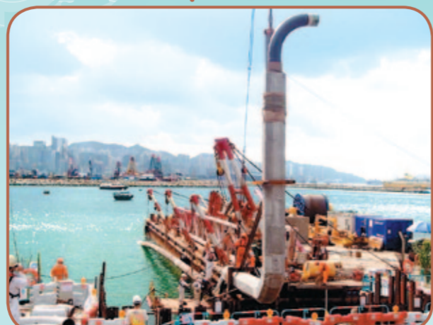
鋪設海底管道工程 Works of laying submarine pipelines
