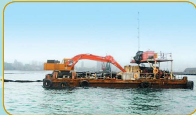
疏浚工程前安裝泥幕 Installation of silt curtain before dredging
